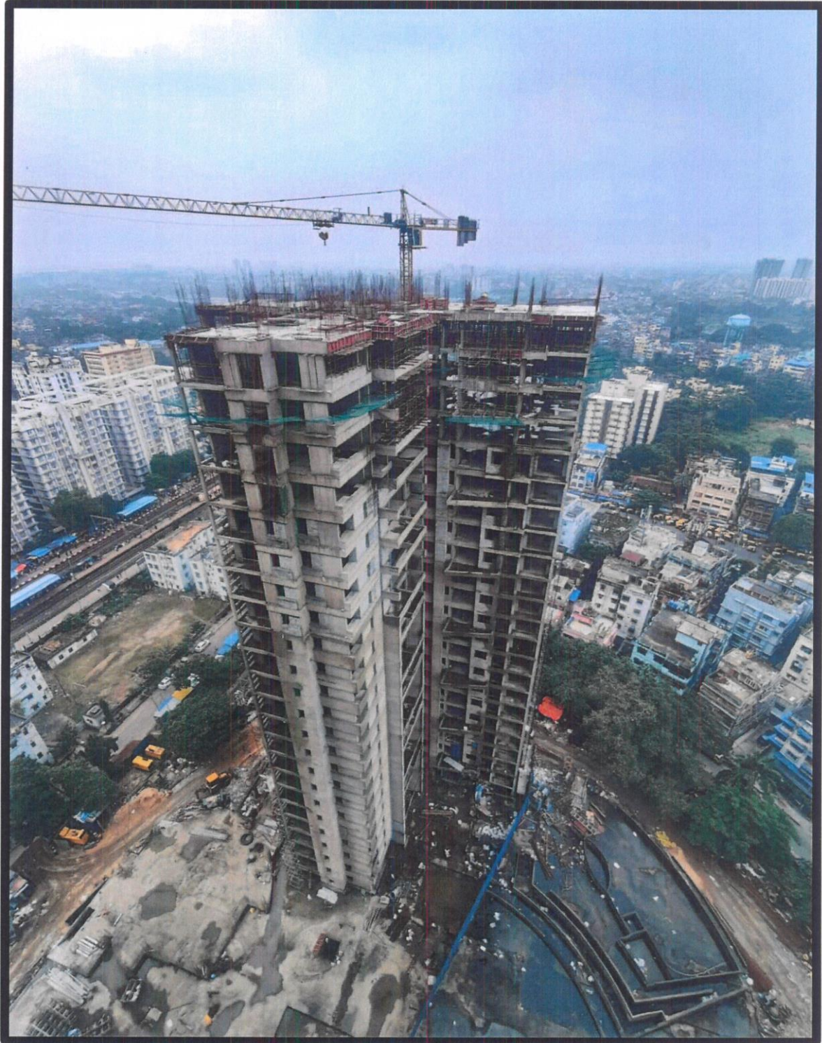
23 rd floor roof casting – Sadashiva Tower
